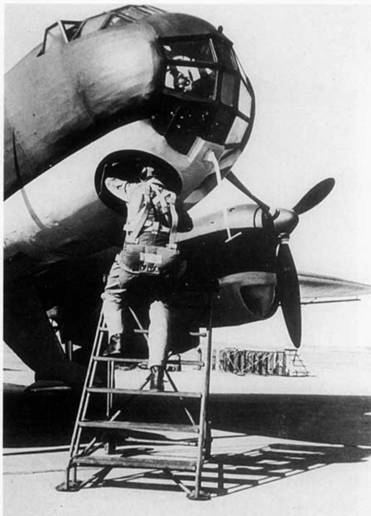
Above: Entry into the pressurized cockpit could only be accomplished by means of a ladder.
